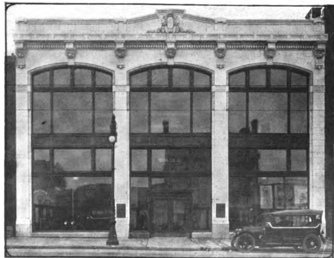
New building of the Longstreth Motor Car Company, Philadelphia, Pa. The structure is of concrete with a terra cotta front. It occupies a space 65 by 125 feet and has a total floor-space of 24,375 square feet. The Longstreth company handles the Alco in Philadelphia and vicinity.
